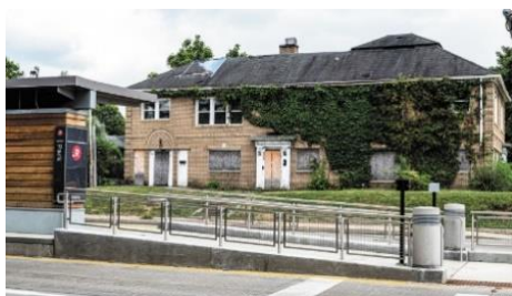
The Broadway Apartments (above left) will replace an abandoned apartment building (below left) across from the Park Purple Line / Red Line Station.
