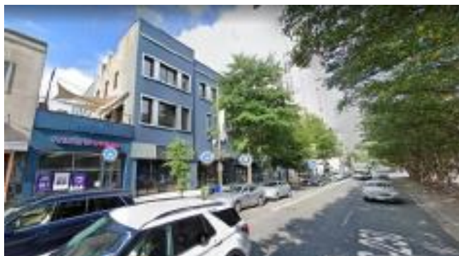
The Gather Arts District promotes its convenience to the Pulse BRT Line on its website (above). The project before redevelopment is shown right; the completed project is shown below.
