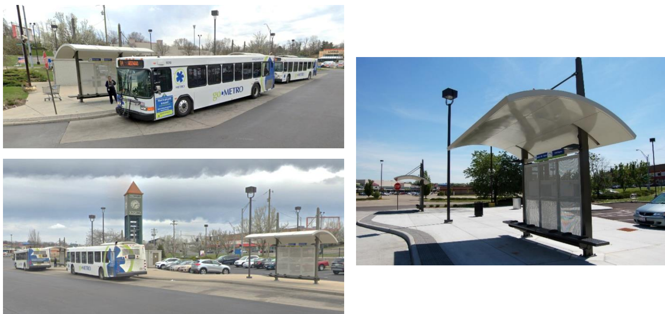
Figure 4-16. Glenway Crossing Transit Center
